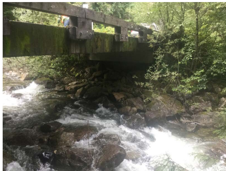
Left Bank Abutment when facing downstream
