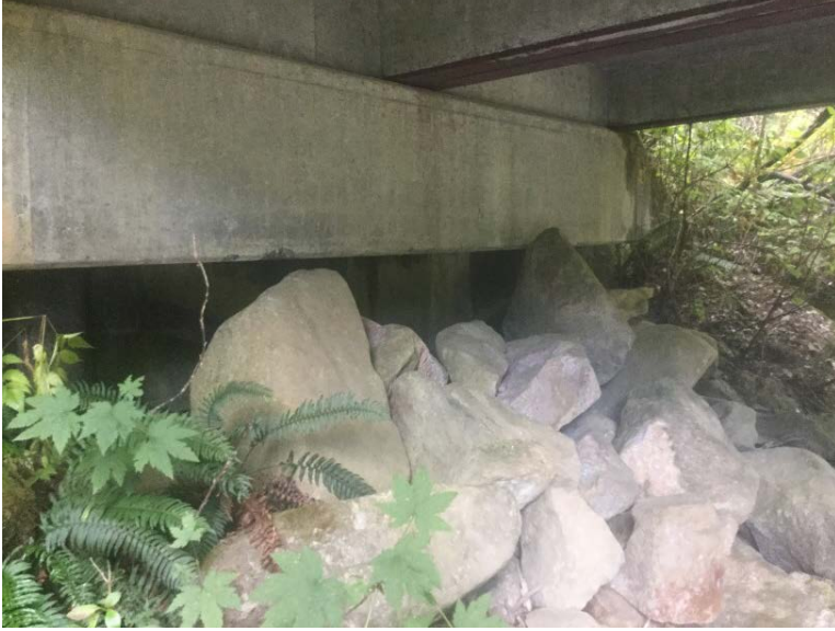
Right Bank Abutment when facing downstream
